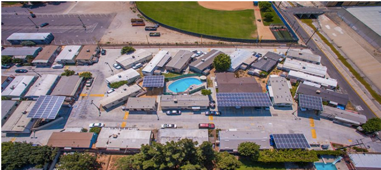
Recent solar development in Compton, CA. http://shorebreakenergy.com/category/photography
