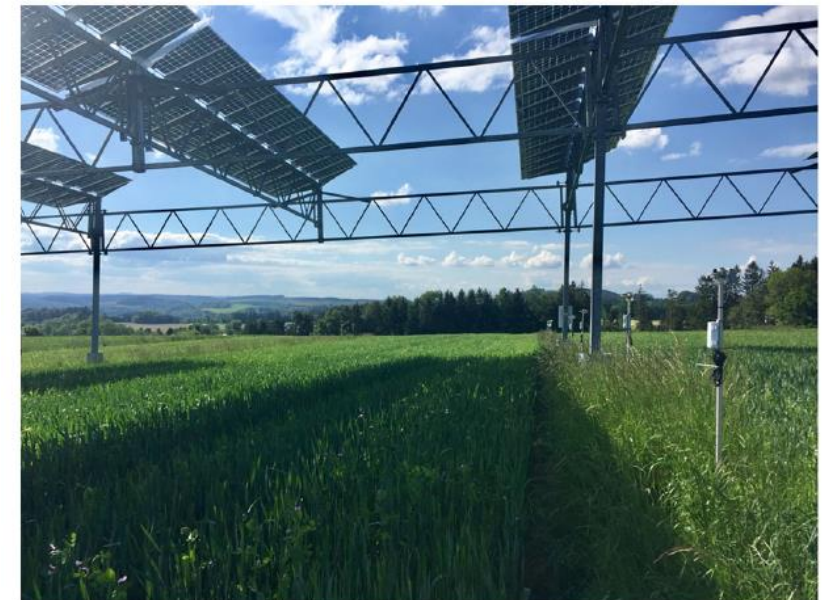
Fig. 1 Shaded winter wheat in an agrivoltaic system in Germany (Photograph by Lisa Pataczek).
